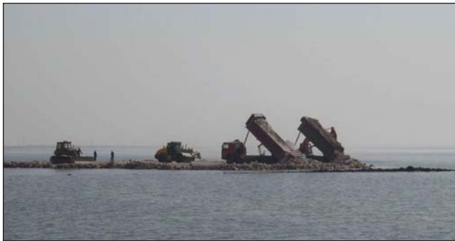
The road being built in the salt ponds. Photo: Bob Loos
