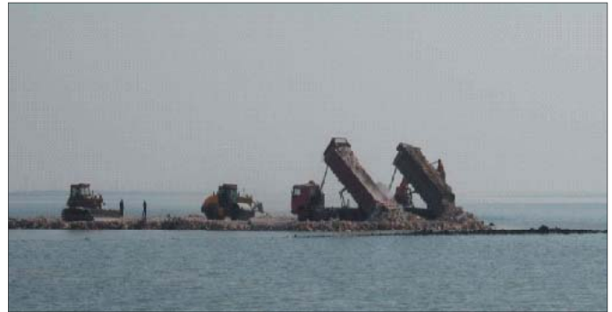
Road building in salt ponds in Bohai Bay. Photo Bob Loos
