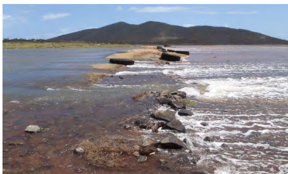
Figure 7. Tidal flows from the estuary zone into the saltpan zone through breaches in the western bund wall during a spring tide in December 2012. (by ©Penn Lloyd)
